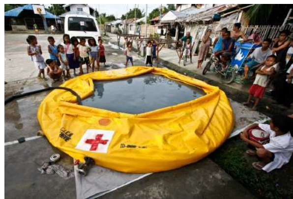
ERU Watsan Iloilo City Philippines Filling up an onion tank with raw water from a well in San Isidro, Iloilo, Panay Island.
